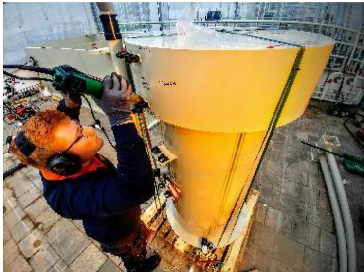
*Figure 2: the DeSludge reactor being prepared for installation in early 2019.*
